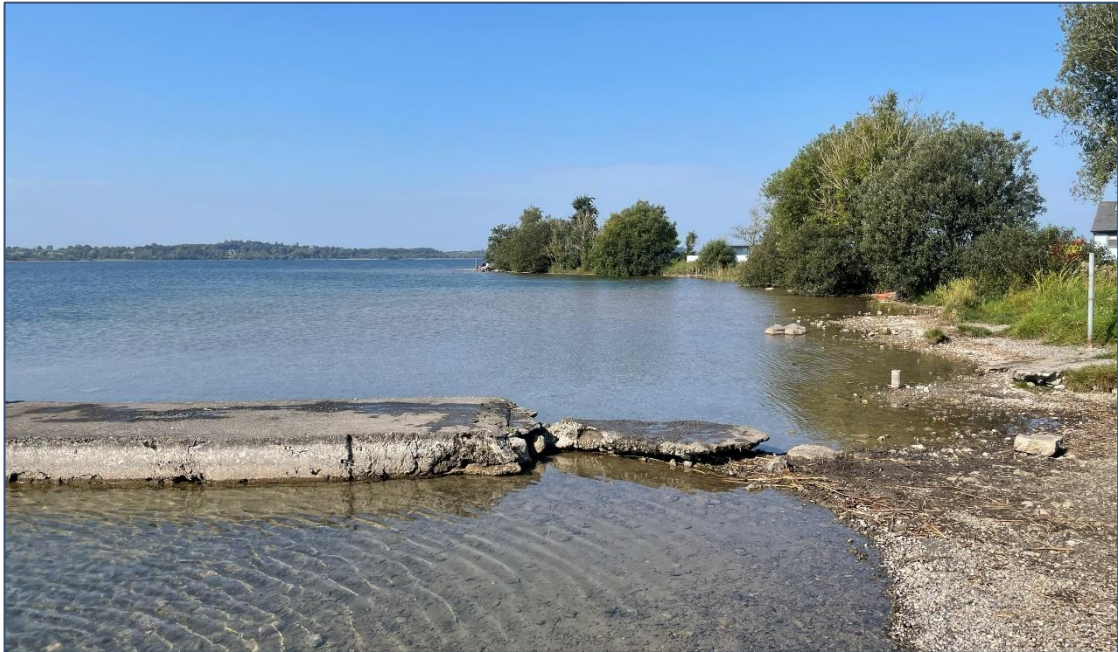
Plate 4: Existing Slipway to be Upgraded
