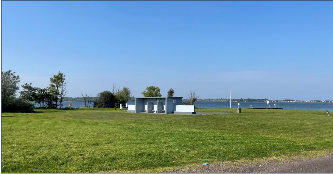
Plate 3: Existing Open Changing Shelter to be Demolished
