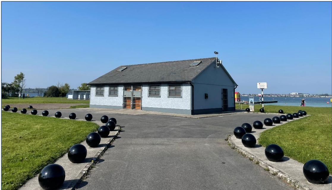
Plate 2: Existing Building to be Refurbished
