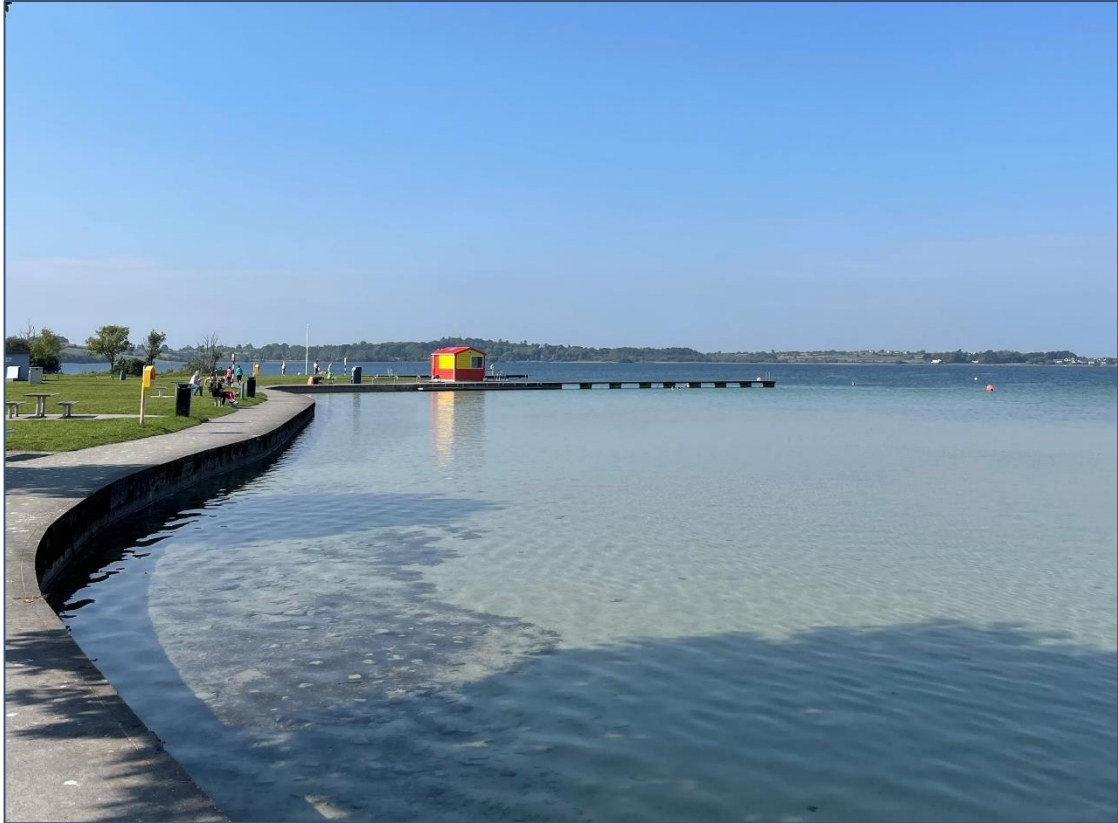
Plate 1: Existing Lifeguard Hut to be Replaced and Pier to be Repaired
