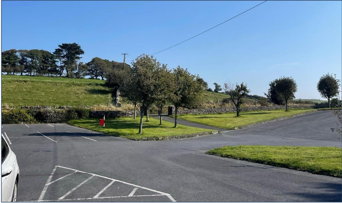
Plate 7: Existing Entrance to be Upgraded
